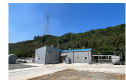
Daesan Plant Wastewater Treatment Facilities
